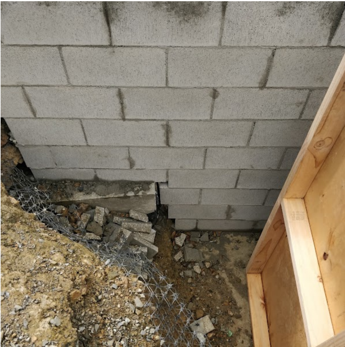
29/11/2021 10:06:11 AMBlockwork transitions - to be boxed out during pour
