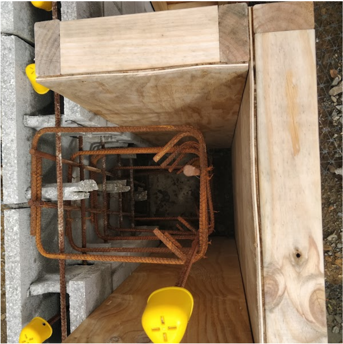
29/11/2021 10:00:00 AM Masonry column bars - as per plan
