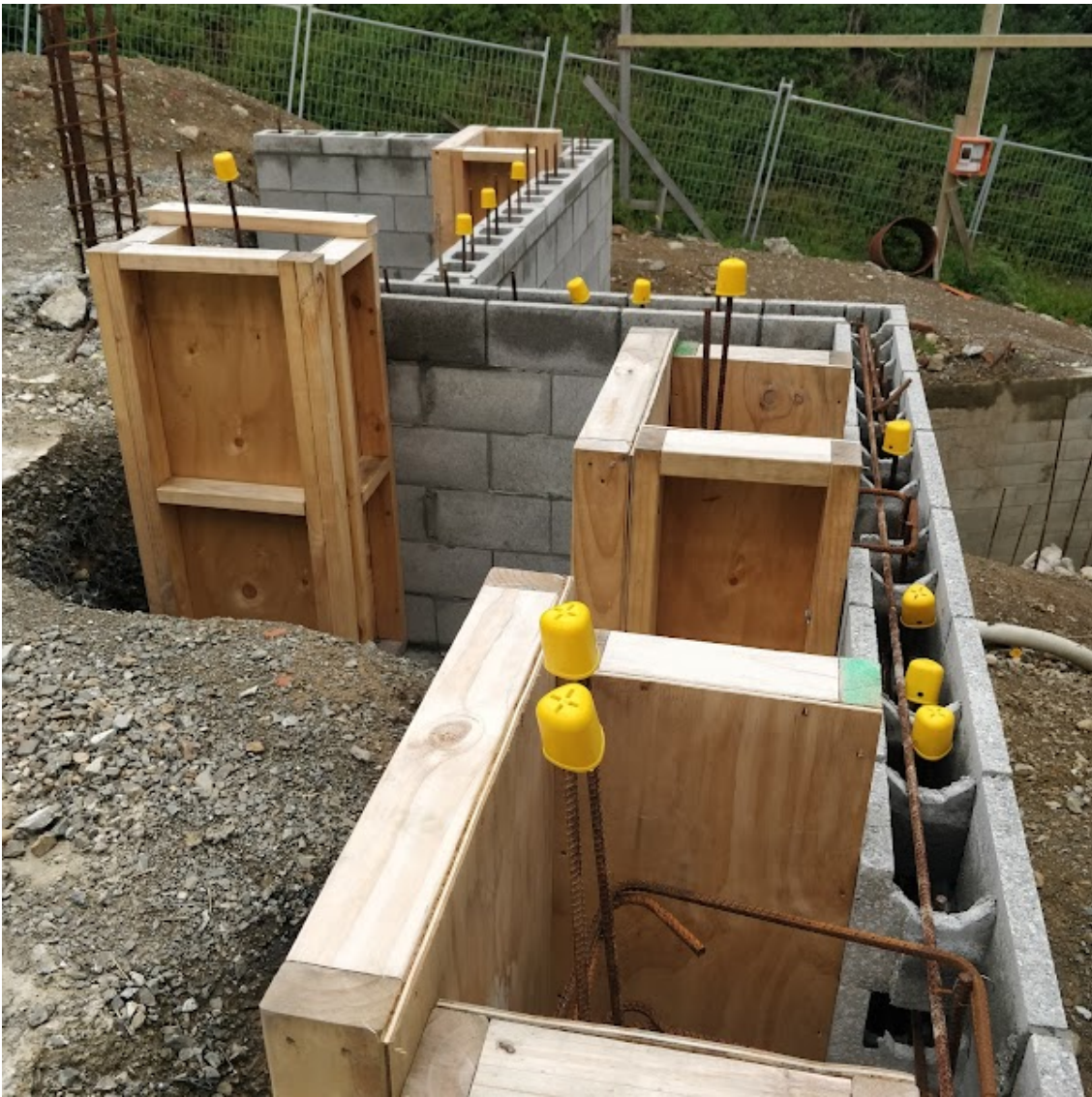
30/11/2021 10:00:00 AMBlockwall masonry column - location as per plan
